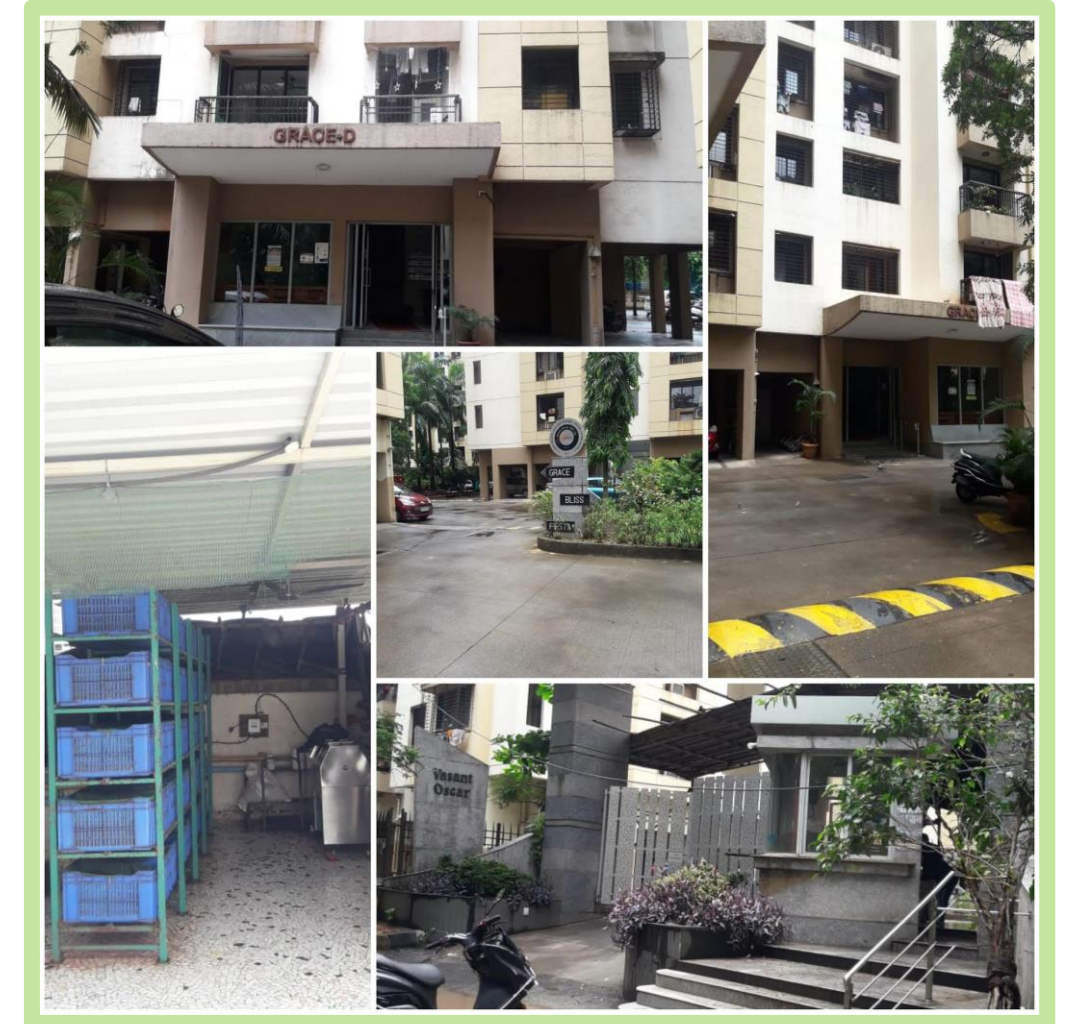
Project Installed On Terrace At Grace Vasant Oscar, Mulund
